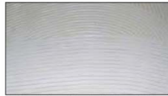
Example of properly troweled adhesive application
